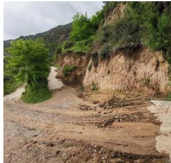
Figure 5. Road subsidence and exposed sliding surface (Point b in Fig.2)
