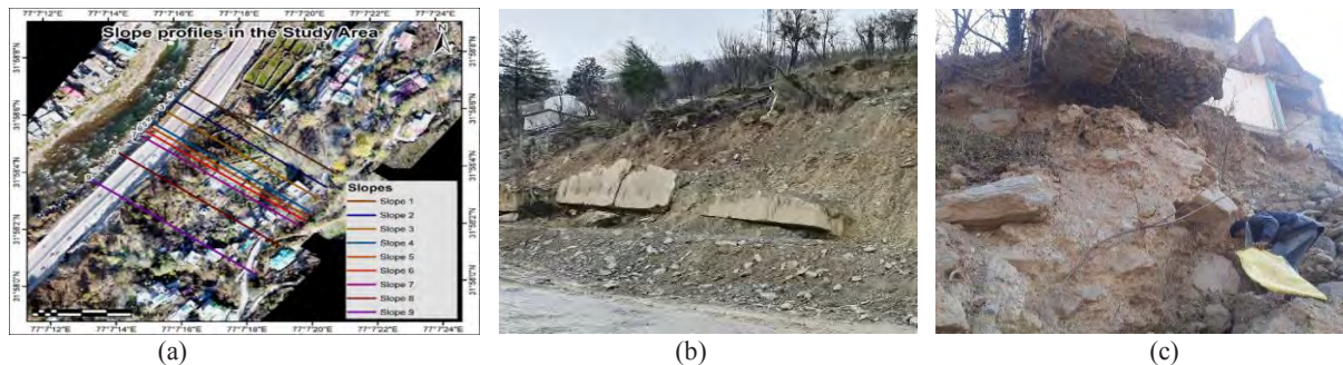
Figure 1: (a) Study area and slope profiles; (b) Failed retaining wall; (c) Exposed foundation of a house uphill
