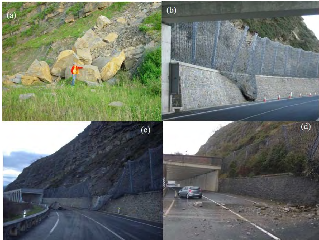
Figure 4. (a) unreported event, retained on top of the gallery, approximately in 2007; (b) reported event on 13/02/2007, without reaching the roadway; (c) event that destroyed the barrier on 02/02/2009; (d) event causing an accident that occurred on 16/11/2019, with much of the volume retained by the flexible barrier. Images b, c, and d, were provided by DFG and Ikerlur).
