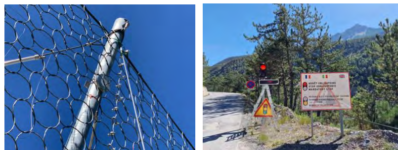
Figure 6: Alerting system installed on 5000 kJ barrier (left). Connection of the alerting system with sign and light on the road (right).
