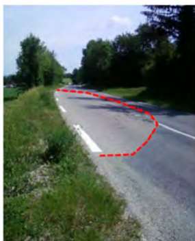
Figure 1. View of surface cracks of the road
