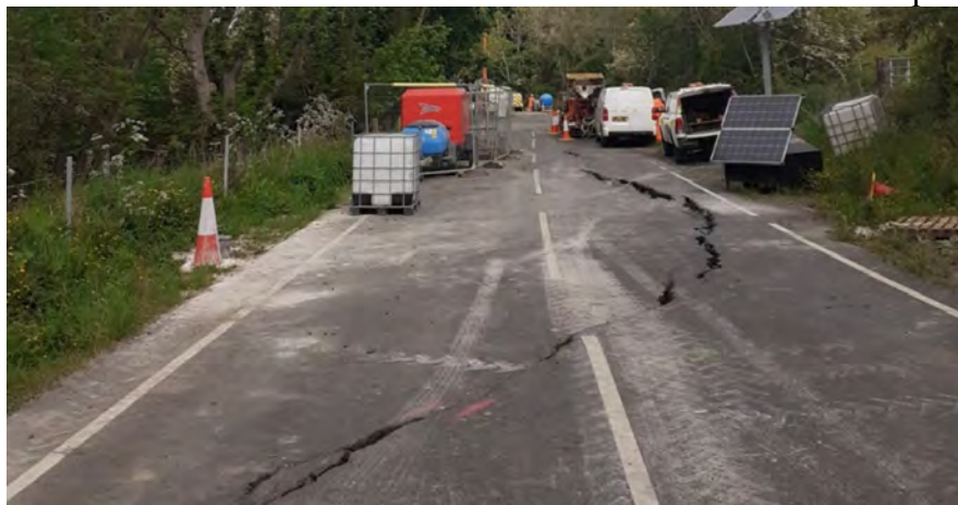
Figure 1. Arcuate cracking within the B6344 following site works
