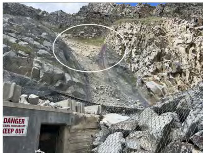
Figure 5. Attenuator mesh on ground after buckling of mid-canyon support post.
