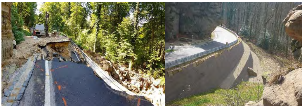
Figure 4. Situation before and after stabilisation
