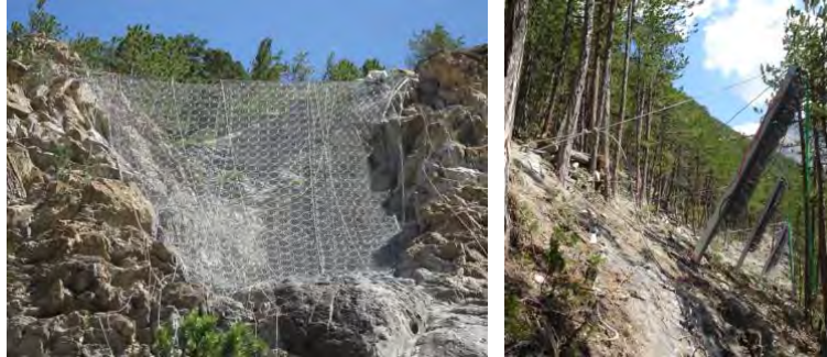
Figure 3: Attenuator barrier (left). Installation of RB 3000 WGC rockfall barrier without anchors at the base of the posts (right).
