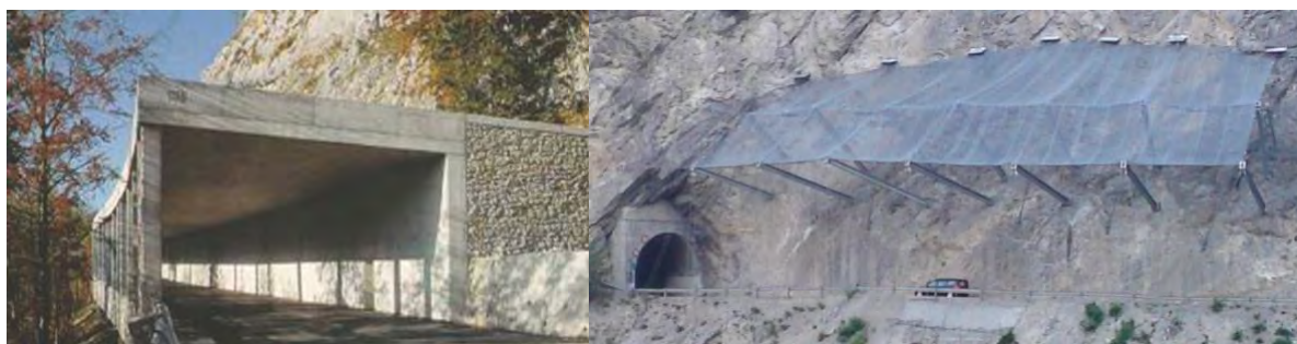
Figure 1: Massive concrete gallery (left) versus flexible rockfall gallery- termed canopy (right).
