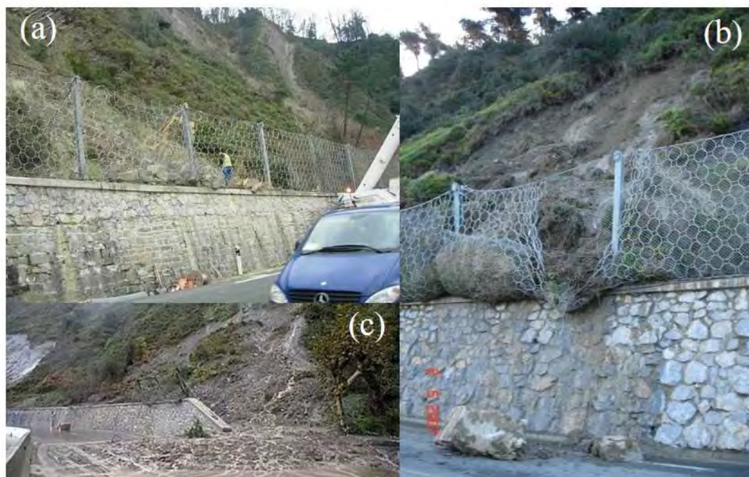
Figure 5. (a) event mostly retained by the barriers that occurred on 02/28/2006; (b) event reported on 05/01/2007, that although the barrier was destroyed, only a minor fraction of the debris reached the roadway; (c) event that occurred on 11/05/2011 in which the debris flow partially bypassed the wall. Images by DFG.
