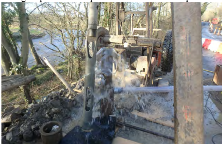
Figure 2. An artesian groundwater strike during the 2016 GI
