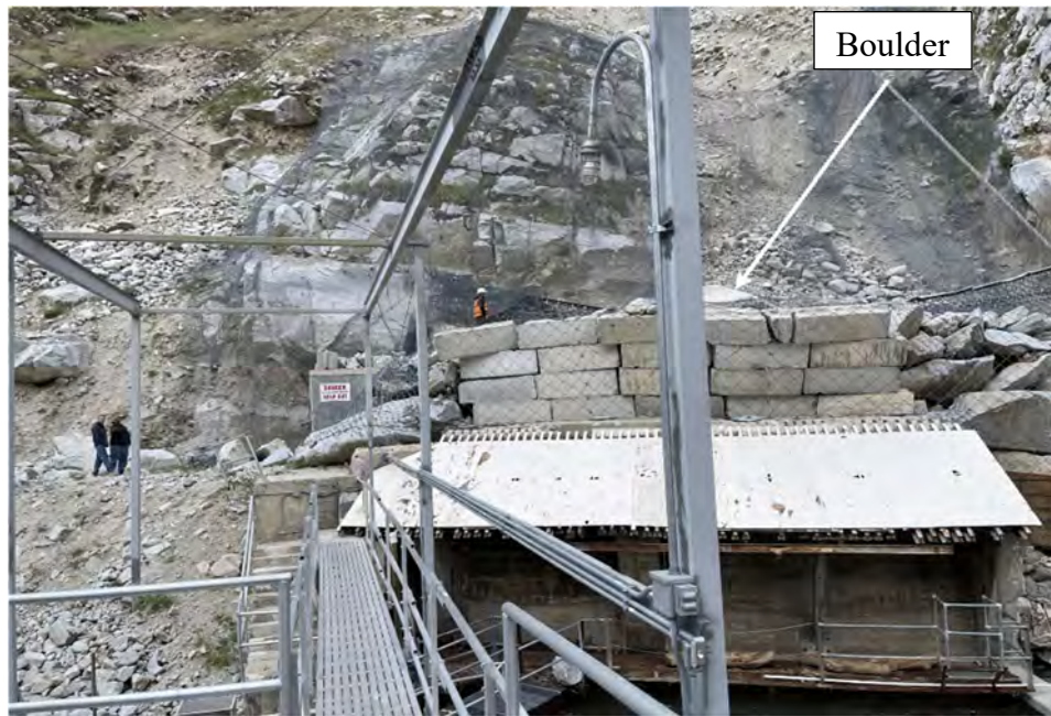
Figure 7. Large 6-m boulder impacted on top of berm.
