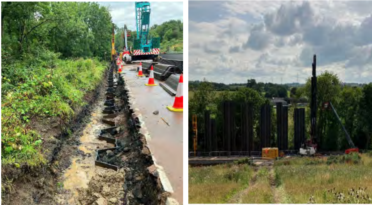
Figure 4. Construction of the Z52 sheet pile wall with rigs advancing behind the wall as a temporary works measure
