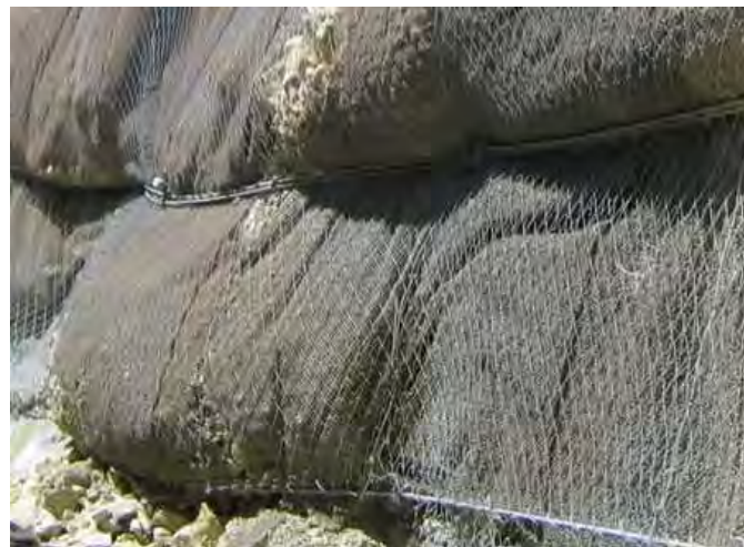
Figure 1 Example of wide punch displacement of flexible structural facing loaded by the soil. The cables reduced the mesh displacement.
